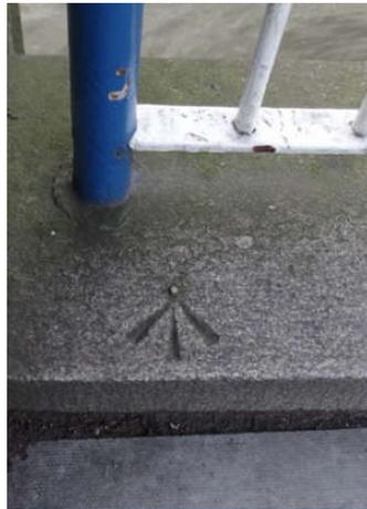
The final example is a flush bracket. It is a G series which means post 1936; G series are found only on walls, never on triangulation pillars. The Bench Mark Database <http://www.bench-marks.org.uk> lists 54 sub-FBs within 2 km of our meeting place at All Saints', including one on the church itself. I challenge you to find it and identify the type on your next visit.
